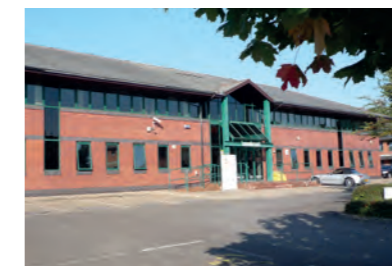
MotoNovo House, Cardiff Business Park
