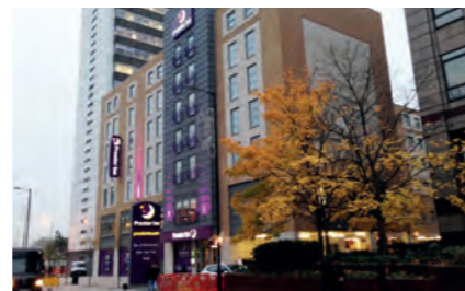
Premier Inn, Lansdowne Road, Croydon
