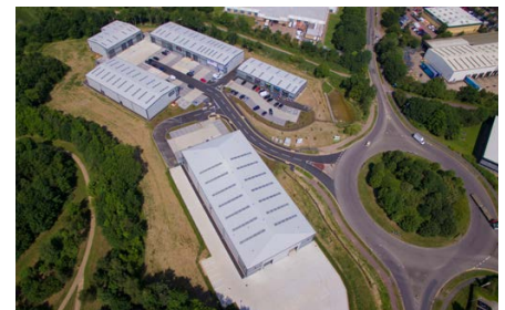
Brackmills Trade Park, Northampton (Industrial)
