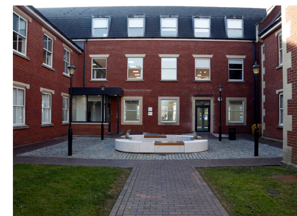
Binsey House, Wallbrook Court, Oxford
