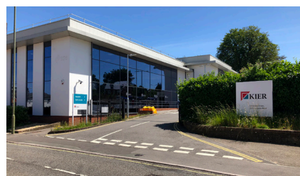
Centenary House, Basingstoke
